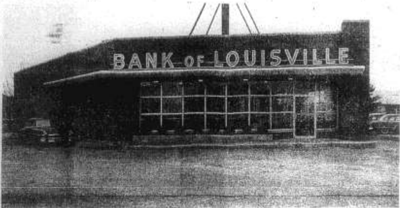
The steadily "open look" of the very modern new St. Matthews office of Bank of Louisville is indicated in this photograph (which was taken before the parking was completed on the drive and parking area). Note car on left at "drive-in" window. The entire building is corded by a yard, so that customers may drive in at the west side and use the east side and transport their banking business without leaving their cars. There is ample parking space in front and rear of the bank for those who prefer to come into the building proper. The almost superlatively good drive-in window is directly east of the Wright bank signs in the park of the country. It has electric light with rear reflector light high, which can be seen for miles a mile along the Shelbyville Road.
